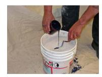
Pour colorant from Tint Pack into "hole" in center of finish.
