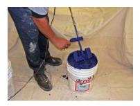
8. Wipe any colorant that may adhere to the blade shaft down and mix until finish color is uniform.
