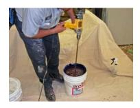
Using a mixer designed for use with EIFS finishes, place blade into finish at bottom of pail. Mix slowly and carefully to ensure all colorant remains in pail.
