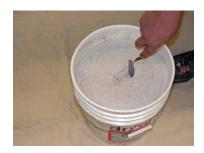
2. Make small "hole" in center of finish.
