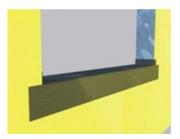
4) Install the AquaFlash System at the jambs in the same manner overlapping onto the sill material a minimum of 2 in (51 mm) – Figure 3.
